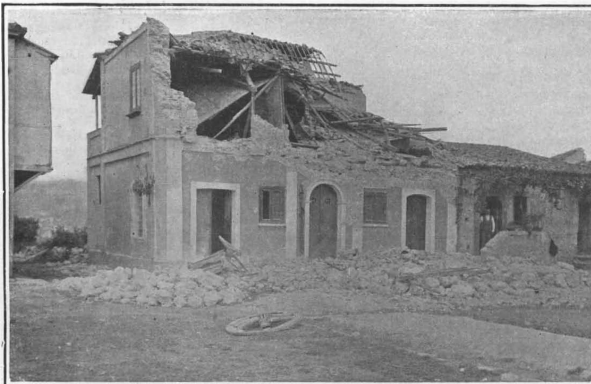
A ruined house near Bagnara.
